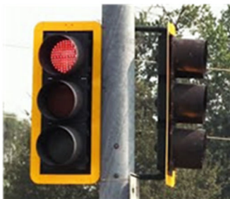
Improve signal hardware: lenses, back-plates with retroreflective borders, mounting, size, and number
