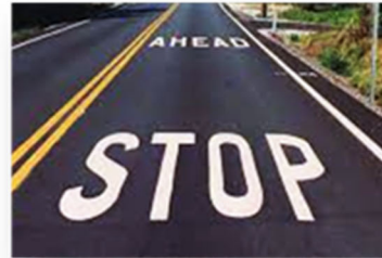
Upgrade intersection pavement markings/ install edge lines
